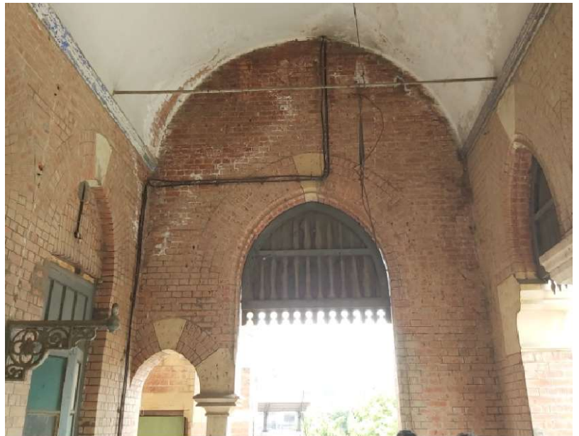
Pointed Arch in brick with Key stone in Sandstone
